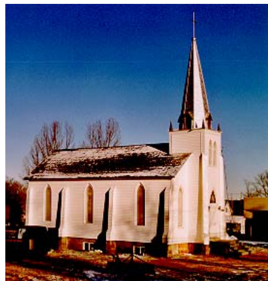
Church of the Ascension on the new foundation.
